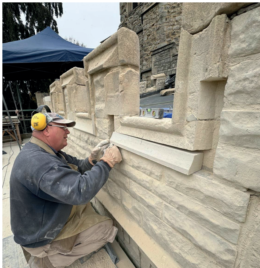
Above: (left): Florian repairs a bronze statue by Gillian Brett on the water fountain in Coronation Gardens in Leyton, East London (Right): Working on a stone indent at All Saints Church in Edmonton, North London
