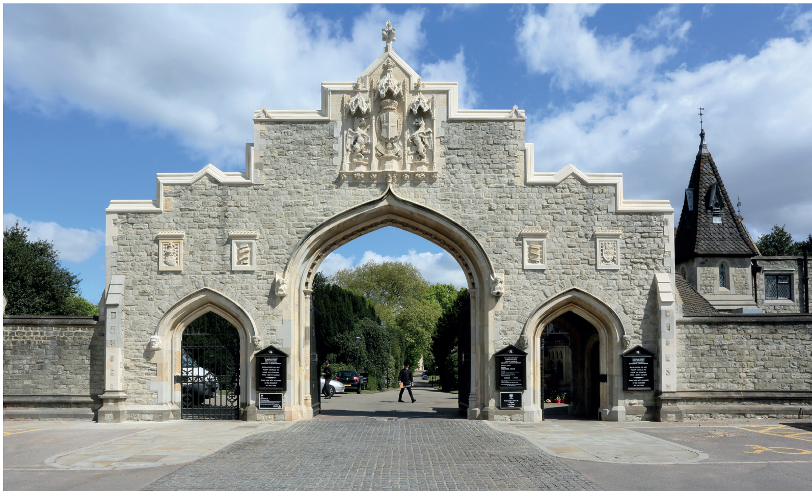
Above: City of London Cemetery. Opposite (top): Site engagement at All Saints Church, Edmonton Opposite: (bottom left): Community engagement at Riversdale Primary School. Opposite (bottom right): Work on Guilford Place drinking fountain
